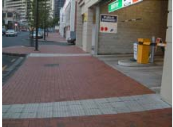
Photo 18: Warning indicators extend across the full width of the footpath outside a car park building.
