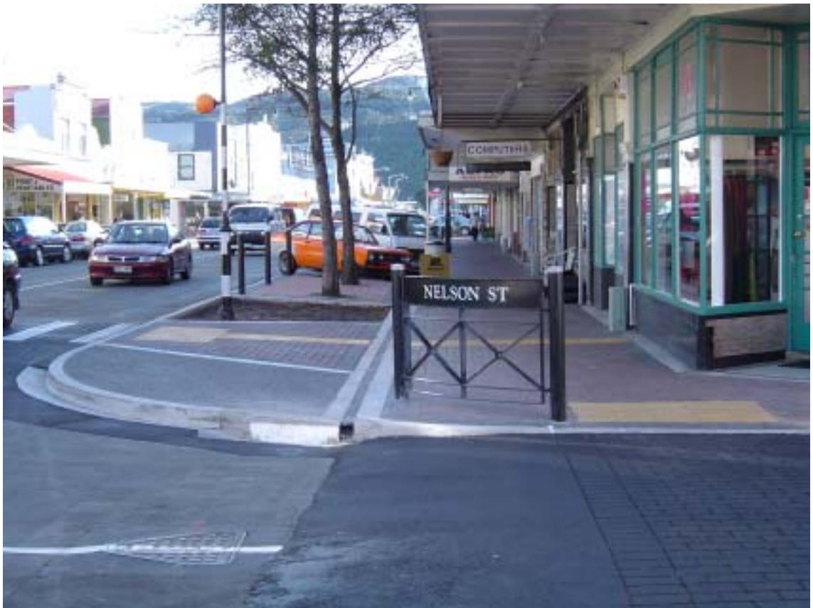
Photo 16: This installation shows a textured and raised crossing surface to inform blind and vision-impaired pedestrians of the boundaries of the crossing point. Note also how street furniture (in this case fencing – with a compliant low level horizontal bar) has been used to divert pedestrians to the crossing point away from the trip hazard at the ramp up to the crossing point.
