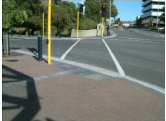
Photo 7: Not good practice: The call box, warning and directional indicators are aligned with the kerb instead of the crossing direction. A blind or vision-impaired person could easily lose their orientation at this intersection and walk into a dangerous situation. There is also poor visual contrast between the TGSIs and surrounding footpath surface.
