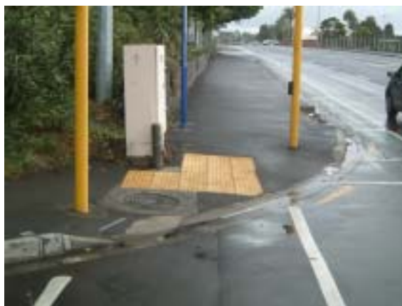
Photo 15: Although not fully compliant, the TGSI convey warning and directional information to blind and vision-impaired pedestrians that encounter them, but it is quite possible to step past them and miss the warning.
