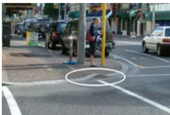
Photo 3: The short kerb upstand between crossing points is a tripping hazard.
