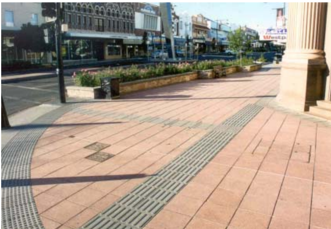
Photo 13: Directional and warning indicators installed at a signalised scramble crossing.
