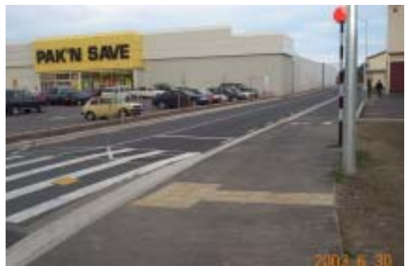
Photo 8: These directional indicators intercept all pedestrians on the continuous accessible path of travel. They lead directly to the warning indicators, which are aligned with the centre of the pedestrian crossing.
