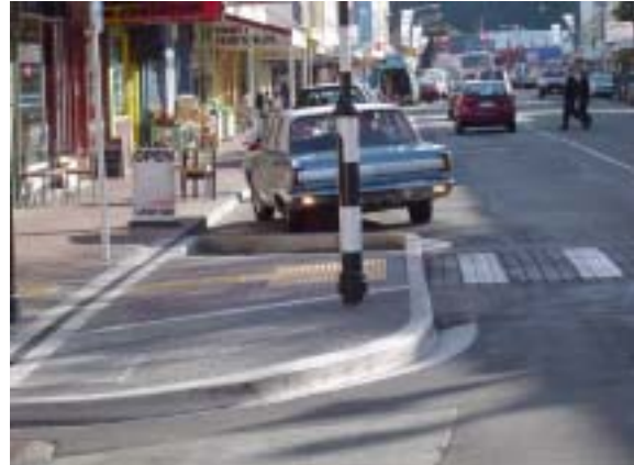
Photo 2: The kerb protrusion at this raised pedestrian crossing reduces the crossing distance for pedestrians. Here a raised crossing slows traffic and eliminates the kerb ramp.
