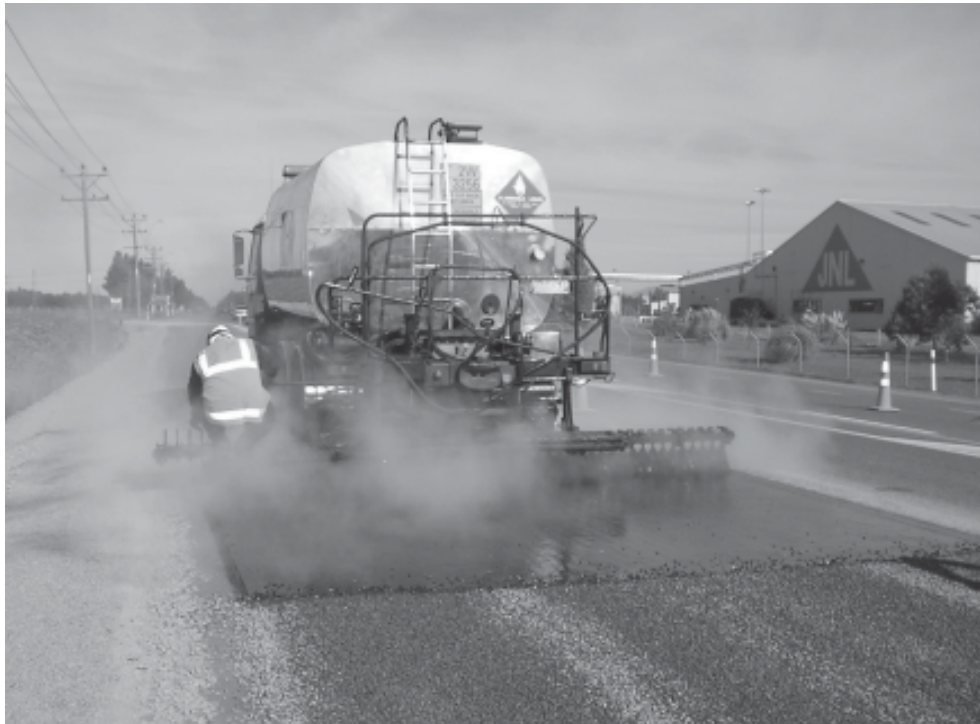
PHOTO: OLDFIELD ASPHALTS
