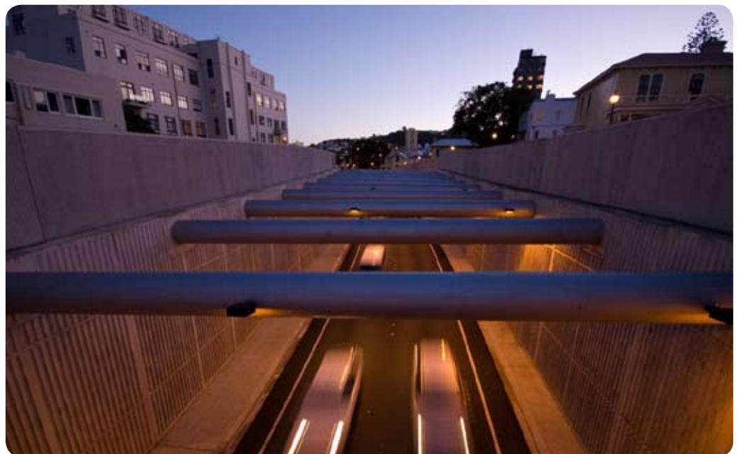
Wellington motorway extension Photo: Stephen Patience
