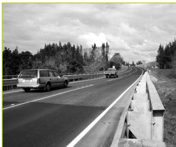
New bridge on SH 1 south of Whangarei. Photo courtesy of Transit.
