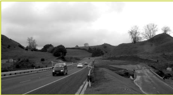
The realignment of the Tapapa curves on SH 5, east of Tirau, will improve safety and travel time on this section of state highway. Photo courtesy of Transit.
